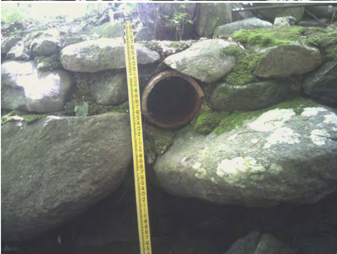
Stormwater outfalls into Deep Brook. Suspected connections to CT DOT Highway Garage.
