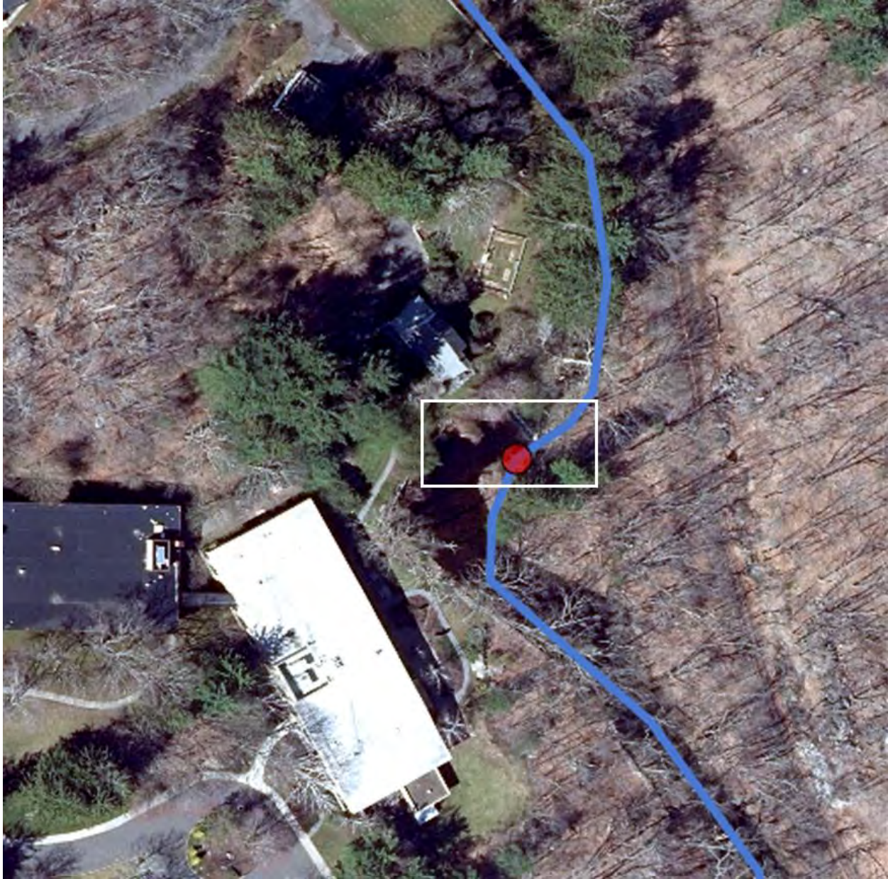
Aerial photo of Deep Brook Dam.
