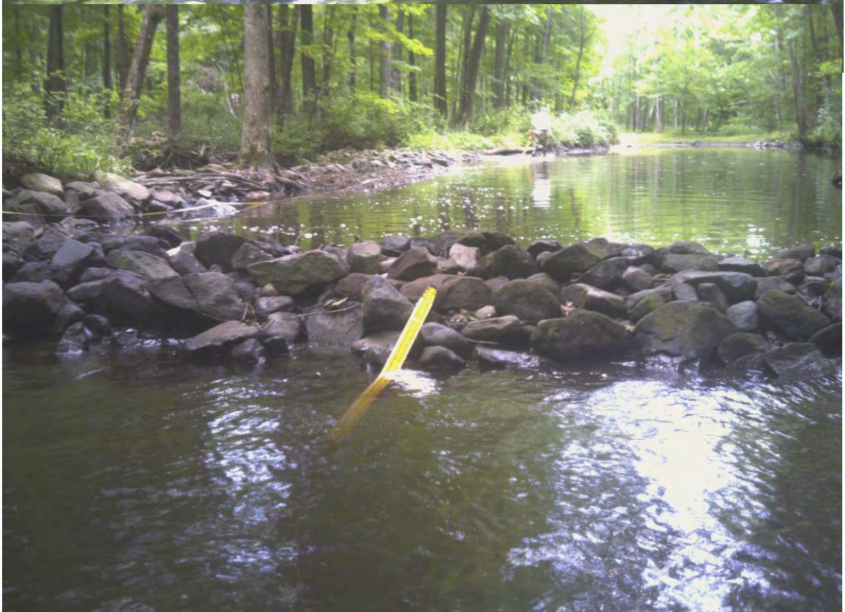
One rock dam in the series of many dams.
